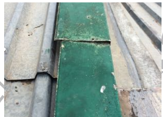
Lapped barge flashing only covering 1 rib and leaking
