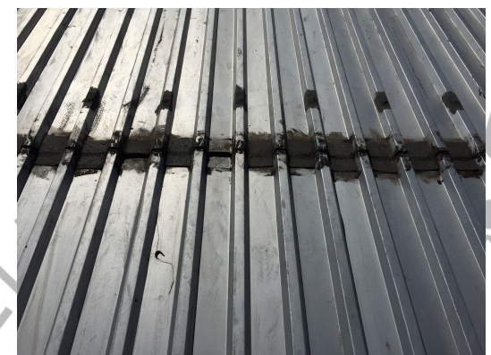
External waterproofing locking the moisture in the lap
