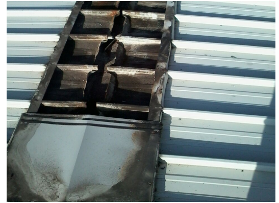
Steel roof sheet material breakdown within the ridge
