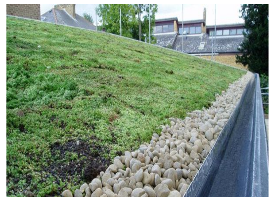
Strip of drainage stones behind retention rail
