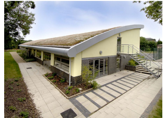
Green Roof on an Aluminum Secret Fix Roof System
