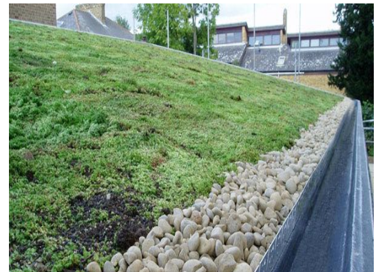
Strip of drainage stones behind retention rail
