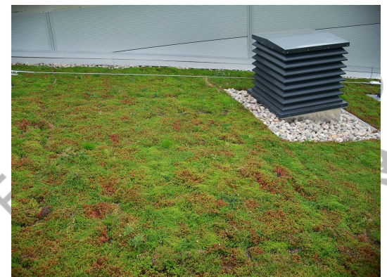
Penetration and drains protected by retention rails
