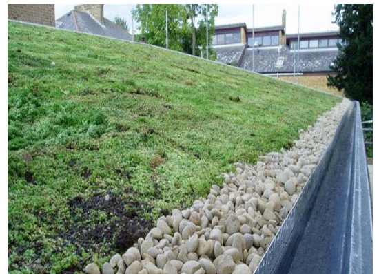
Strip of drainage stones behind retention rail
