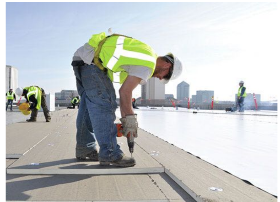
Insulated Single-Ply System mechanically fixed
