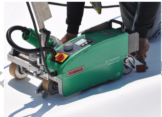
Hot air welding of the Single-Ply Roof Membrane
