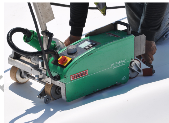
Hot air welding of the Single-Ply Roof Membrane
