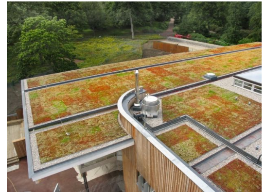
Green Roof on a Single-Ply Roof Membrane System
