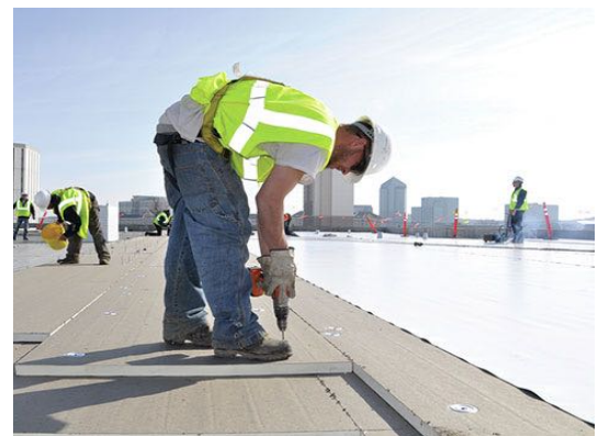
Insulated Single-Ply System mechanically fixed
