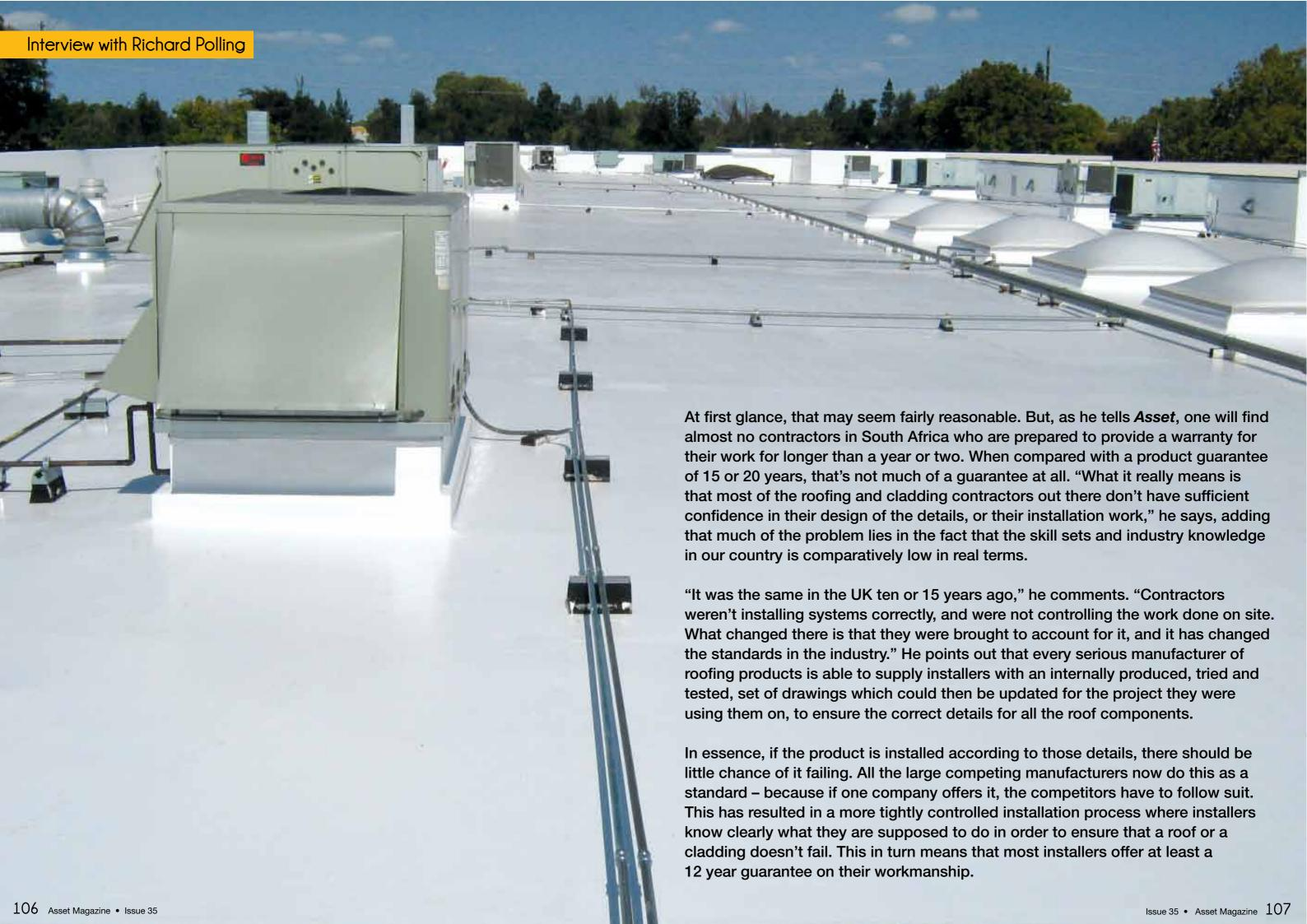
"I always tell people that roof sheets don't leak. If your roof is going to leak or fail, it will be around the perimeter, or around any penetrations," Richard explains. Getting details such as roof ridges, eaves, and flashings correctly designed and constructed is therefore critical to the performance of the installation.
