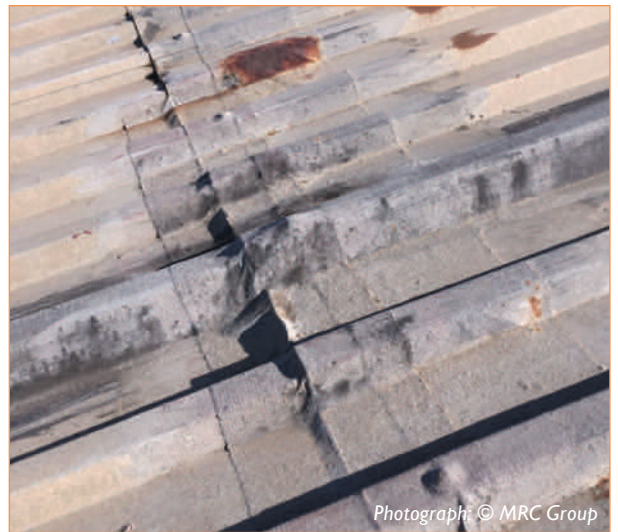
Photograph: © MRC Group Standard waterproofing solution to water leaking through the end lap.
