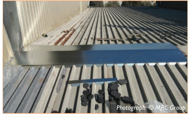
Photograph: © MRC Group Due to the low roof pitch 925mm girth metal ridge flashing complete with serrated closures, polyclosures, sealants and turn-ups in lieu of the standard 462mm girth metal ridge flashing.
