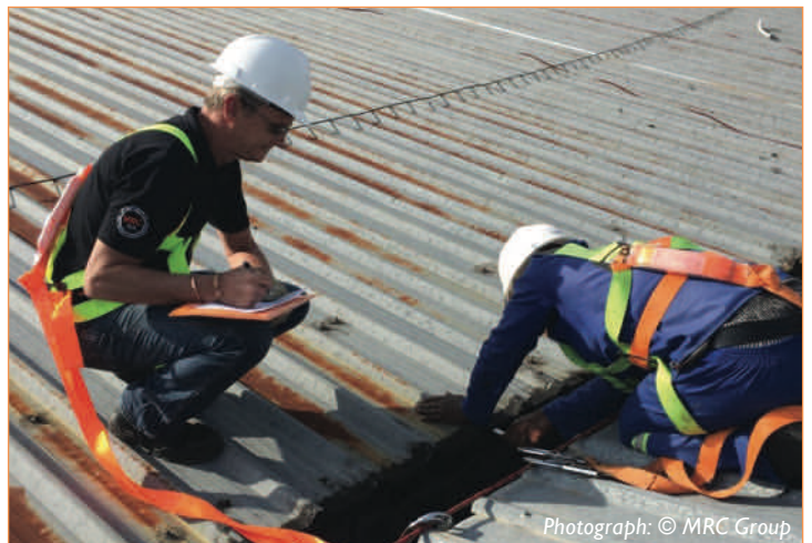
Essential recorded maintenance of the roof system.
