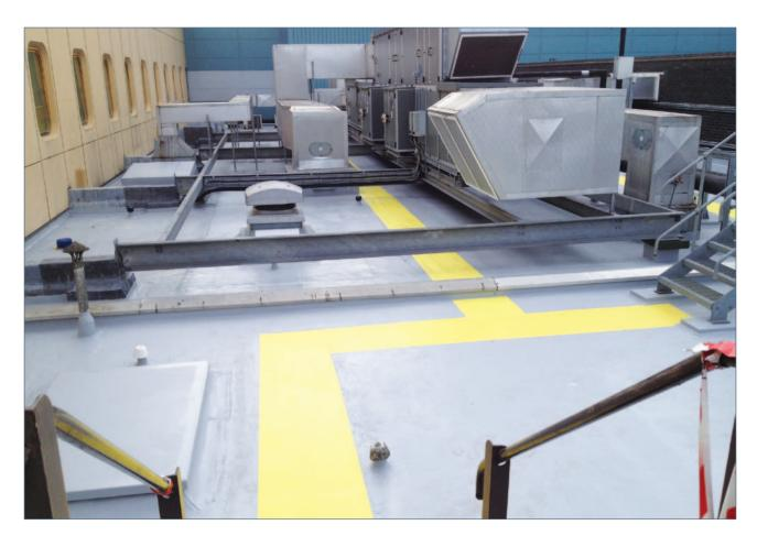
Some products offer great LRV, but the emissivity of the material may be low – often reaching extremely high temperatures of around 80°C. These temperatures increase thermal movement, resulting in preventable damage. For best results, source products that offer a combination of impressive LRV, Emissivity and Solar Reflectance, for a well-rounded waterproofing solution that will extend the life of the roof, reduce energy needs, and ensure no further leaks for many years to come.
