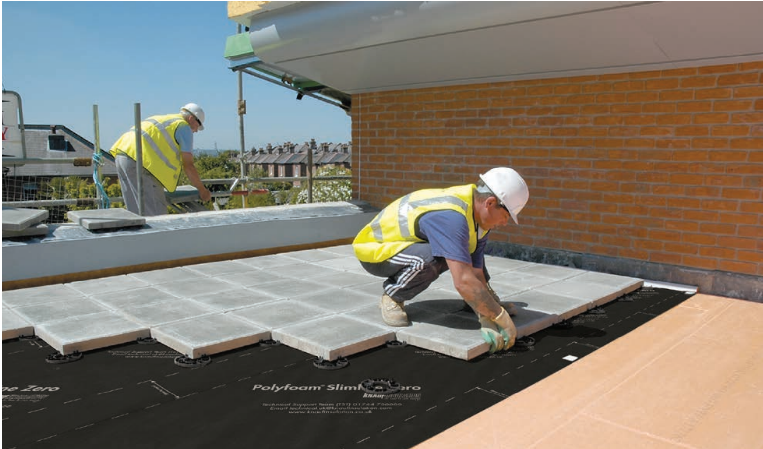
An inverted roof with paving.
