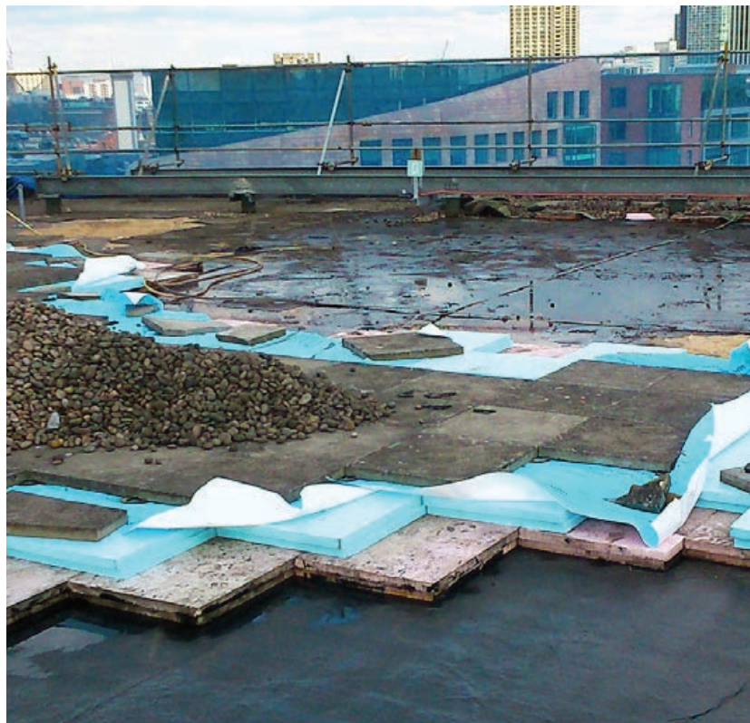
Liquid-applied inverted roof.
