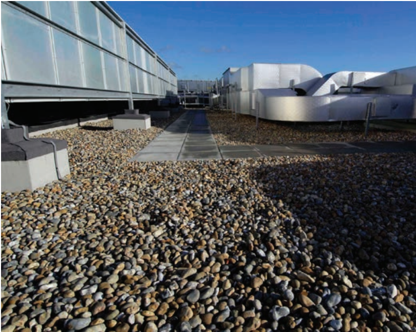
Ballast inverted roof.
