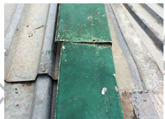
Different size lapped barge flashing causing leaks
