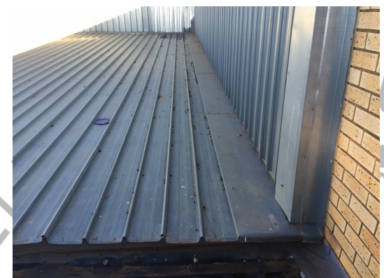
Metal sidewall flashing with vertical cladding
